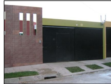
Residencial Villas Arizona $46,632.00
